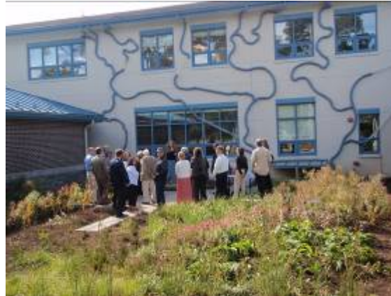
Springside School "Water Wall" and Rain Garden
