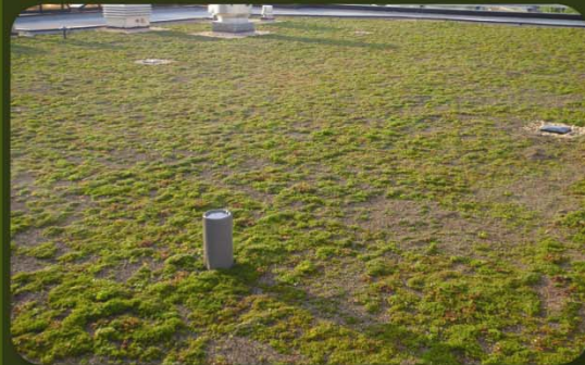
PECO Building, Philadelphia, PA
