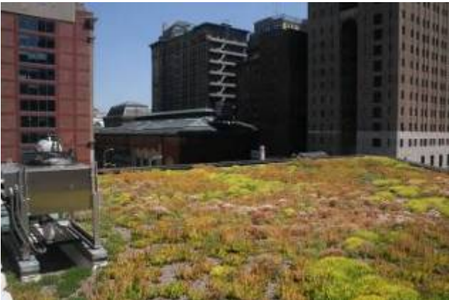
Friends Center Green Roof
