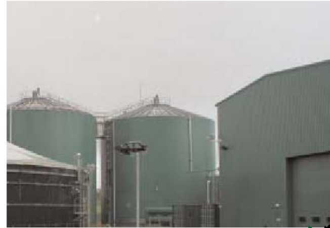
Large scale co-digestion plant, Holsworthy, UK (Picture courtesy of Rudolf Braun, Austria)
