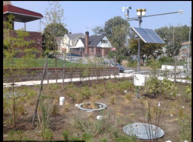
Nashville site: hydraulically connected to surrounding street and sidewalk catchments through curb cut (11:1)
