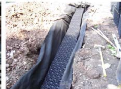
INSTALLATION OF INFILTRATION CHAMBER
