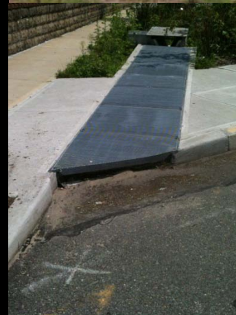
Nashville site: hydraulically connected to surrounding street and sidewalk catchments through curb cut (11:1)
