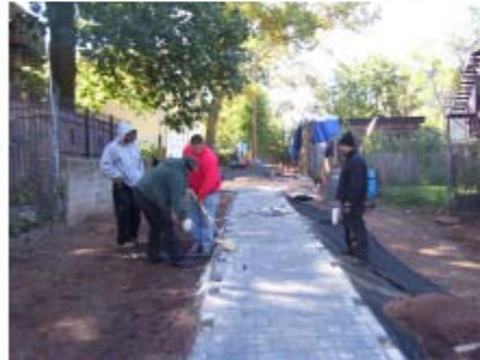
INSTALLATION OF PERMEABLE PAVER WALKWAY
