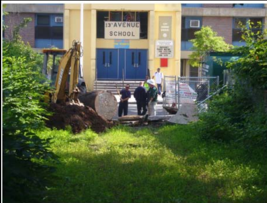
PROJECT SITE - BEFORE
