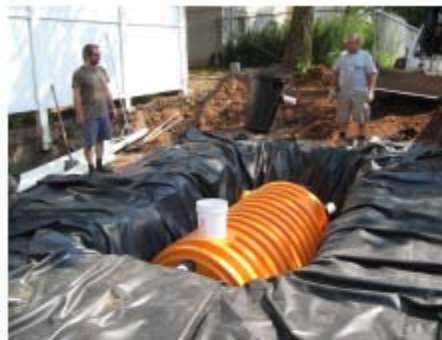
INSTALLATION OF SUBSURFACE CISTERN (AKA STORMCHAMBER)
