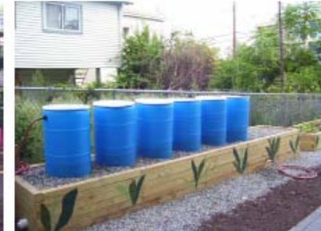
RAIN BARRELS ON RAISED PLATFORM WITH SPIGOT CONNECTION
