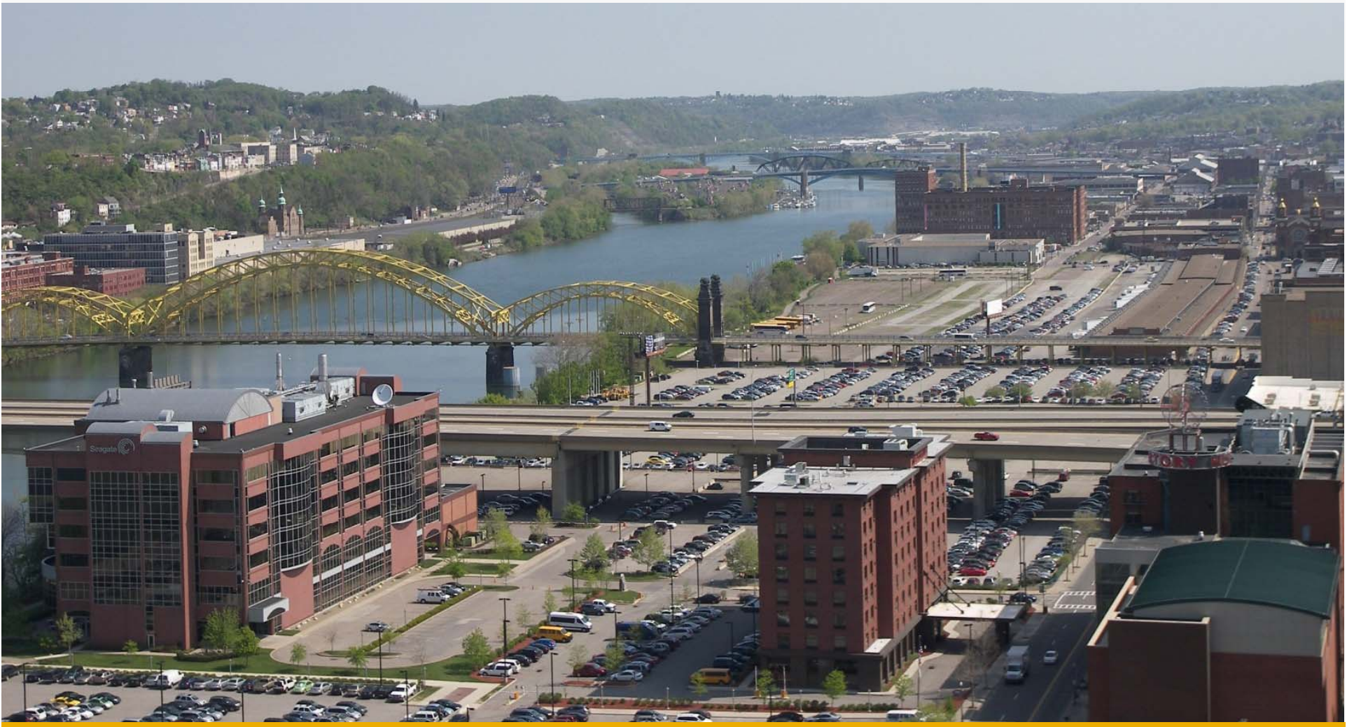
View looking east from 11 th Street
