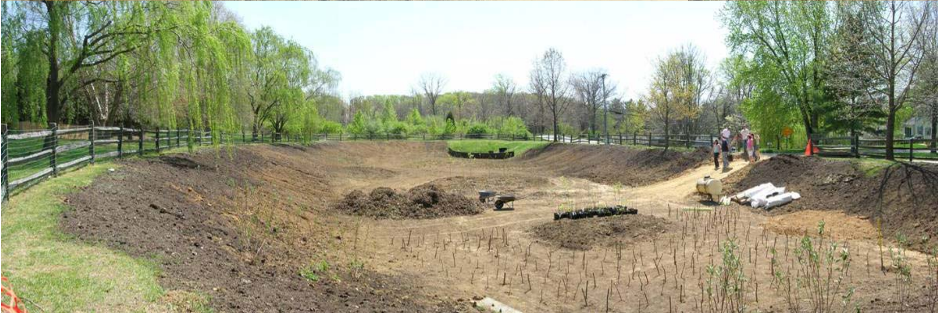
Volunteers planted 300 live stakes and 200 container grown trees and shrubs. After planting the basin was seeded with wet and dry native grass and forb mixes. April 2006
